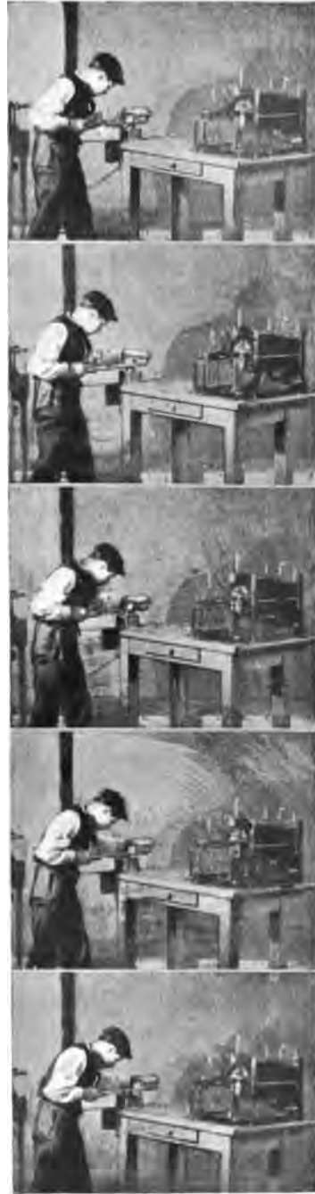
FIG. 66. Apprentice (Fitter) filing Metal. To the left, the Correct Attitude; to the right, the Incorrect. (The Sequence of the Pictures is from Top to Bottom.)
